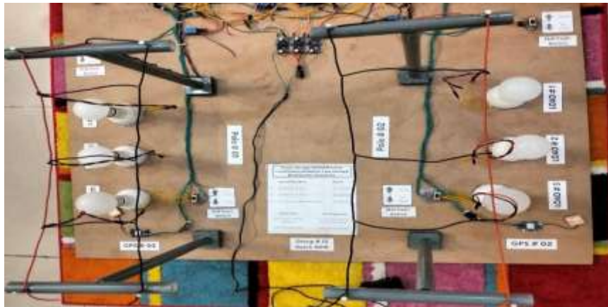
Figure 9: Street Distribution Pole with three 12V,7W AC light bulbs and individual GPS Sensors
